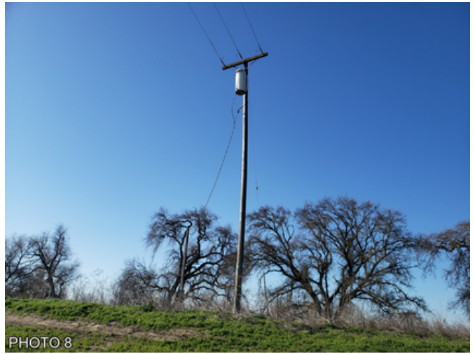
POLE MOUNTED TRANSFORMER
