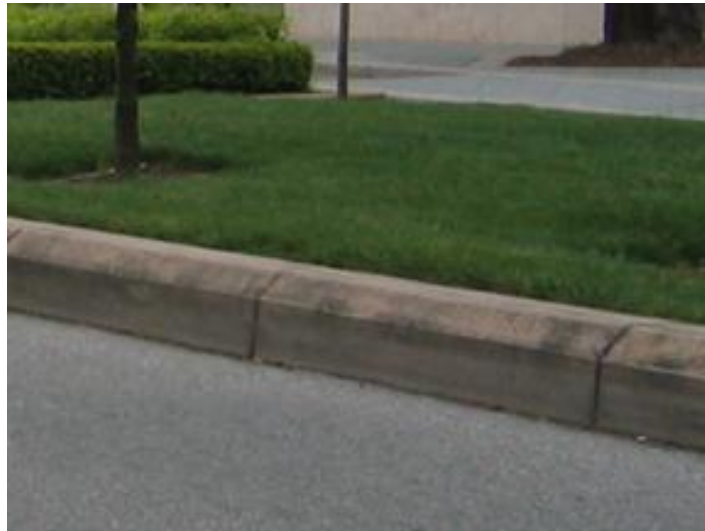
Raised curbing at entry
