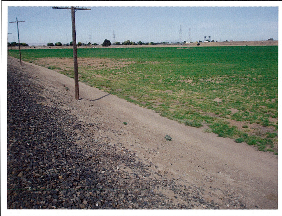
The storm drain alignment follows the base of the elevated railroad tracks; 08/12/09.
