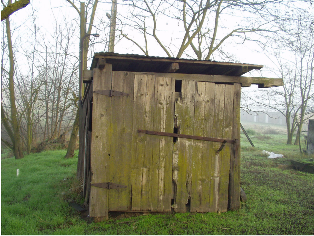
Storage Shed #1 observed in middle portion of Property. View to N.
