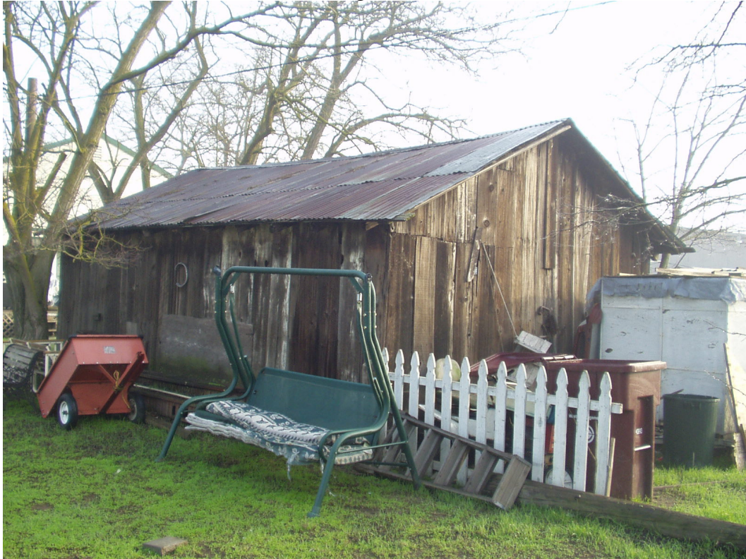
Storage shed #3. View to NE.
