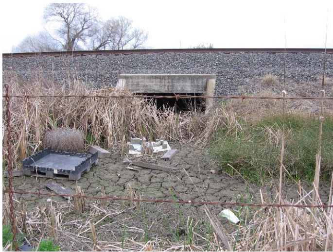
CULVERT FROM POND TO CREEK
