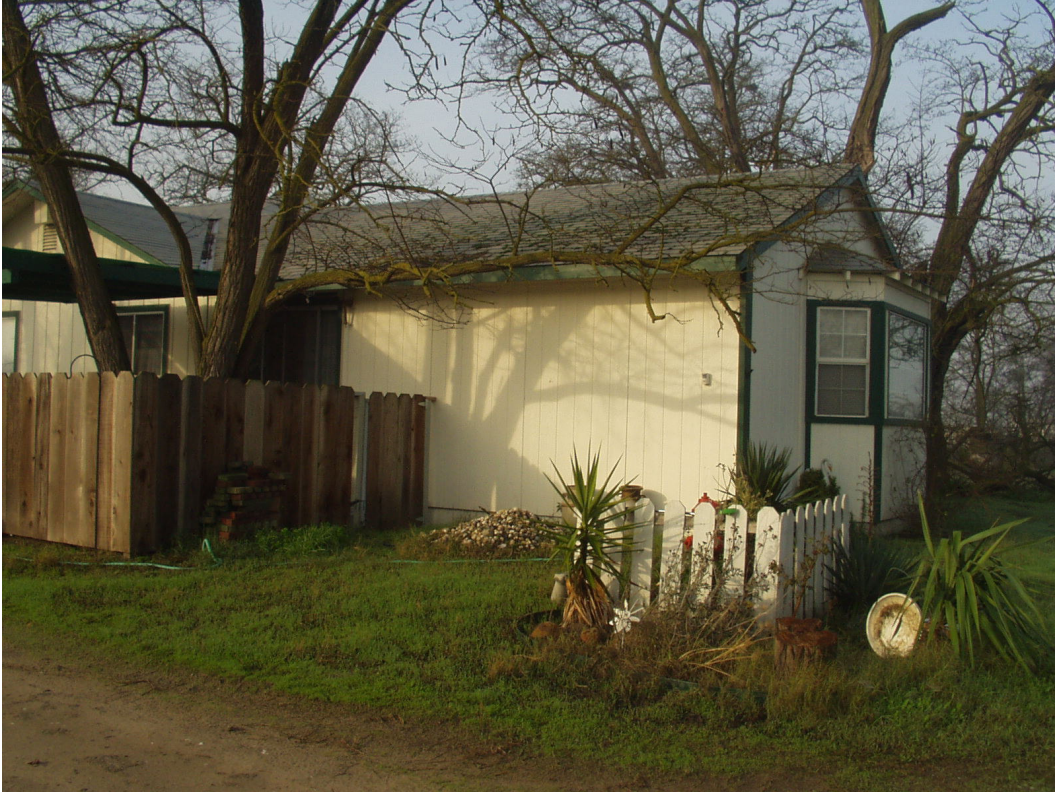
Residence #1. View to W.
