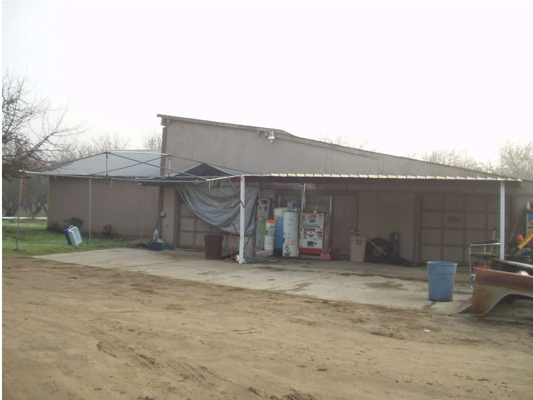
Workshop located in middle portion of Property. View to E.
