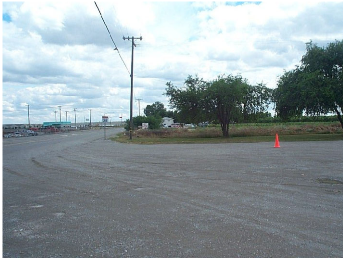
NORTH BOUNDARY LOOKING EAST AT W. YOSEMITE AVENUE
