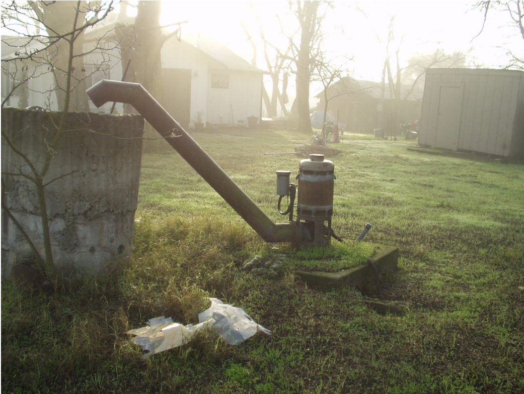
Irrigation well located west of Residence #1. Storage shed #2 and #3 observed in background. View to SE.
