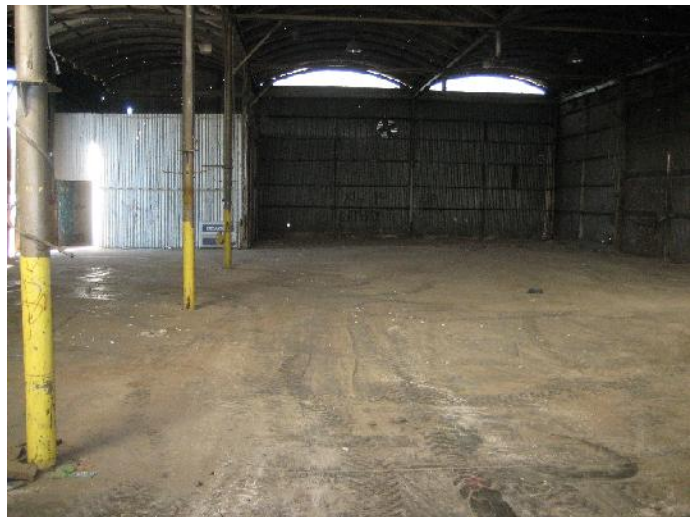
VIEW OF INSIDE OF BARN
