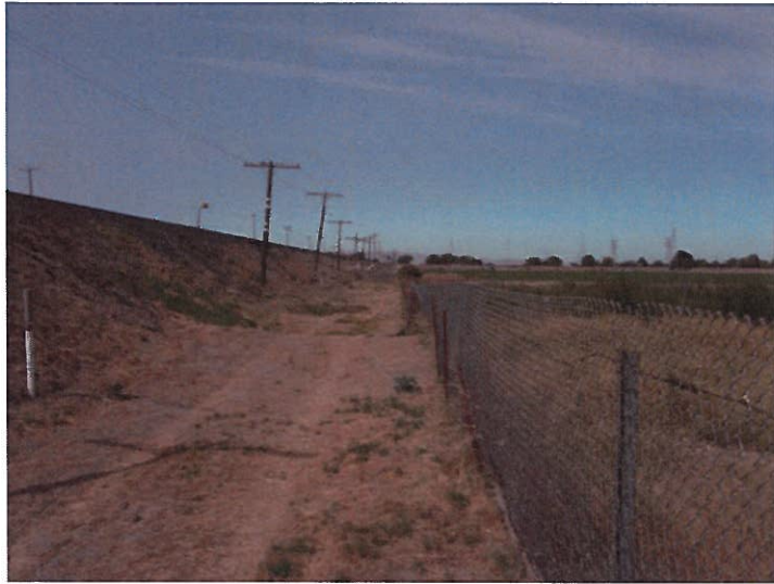
← Look south-west along UPRR right-of-way toward San Joaquin River.
