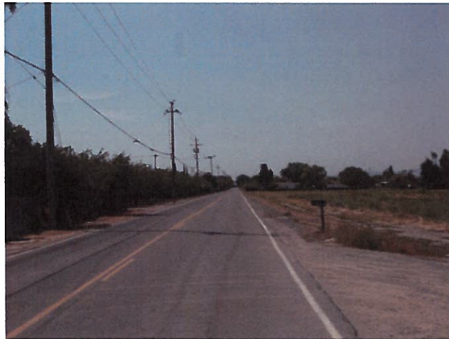
← Looking south along McKinley Avenue from Yosemite Avenue.
