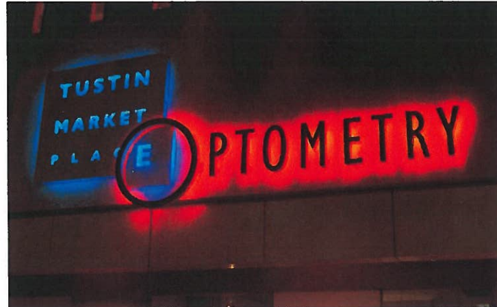
Mixed Media: Halo illuminated channel letters with an aluminum panel routed copy
