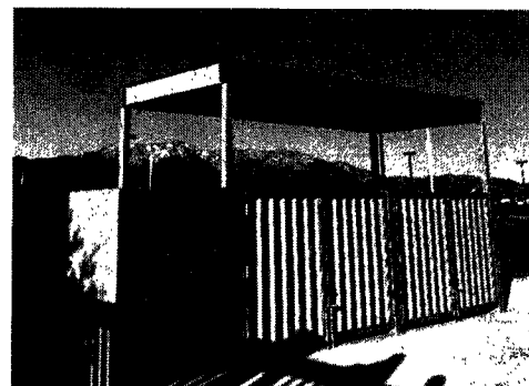
Photo Example 8 Enclosed refuse areas
