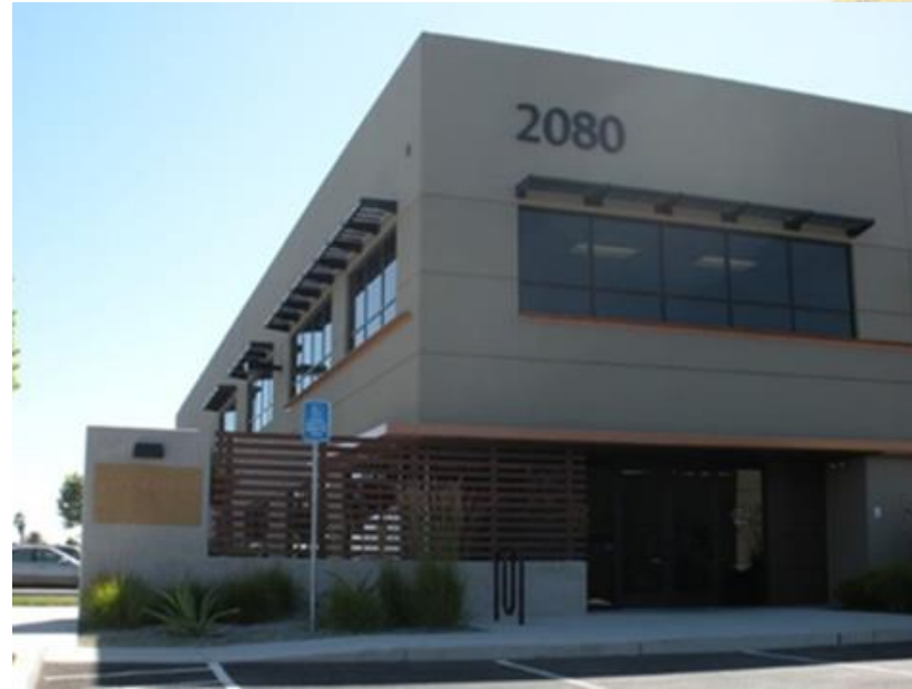
Entry protected from the elements
