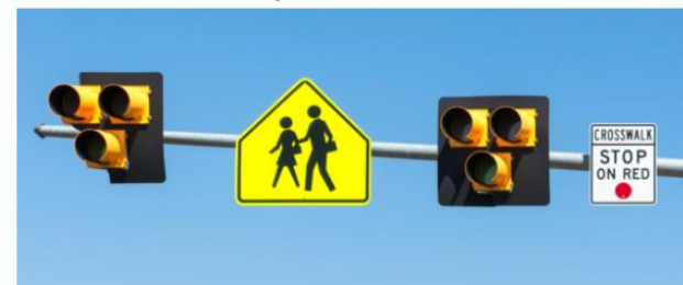
Install Pedestrian Hybrid Beacons
