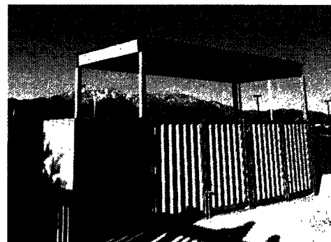
Photo Example 8 Enclosed refuse areas
