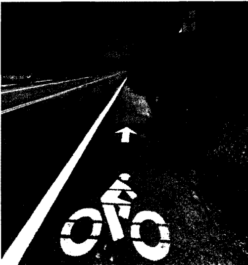
Overgrown vegetation obstructing bicycle facilities can create a hazard and should be kept clear of the path of travel; Source: Bicycling Monterey
