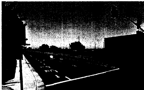
South Harlan Road Class II bicycle lane at J Street, bicycle lane dropped at right turn pocket
