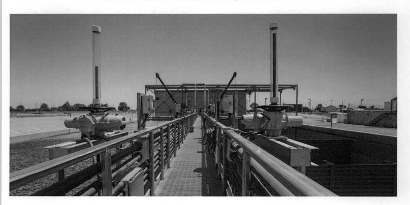
The Phase 4 expansion proposed is based on careful planning and organization established in Phases 2 and 3. The Phase 4 design will include the final headworks expansion, splitting of the inflows to all three pairs of trains, re-combining at the downstream end, new air equipment, and new MBRs.
