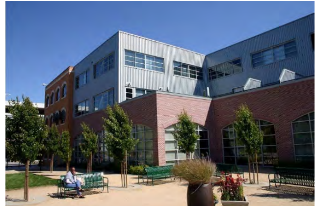
Photo Example 15 Employee well-being area
