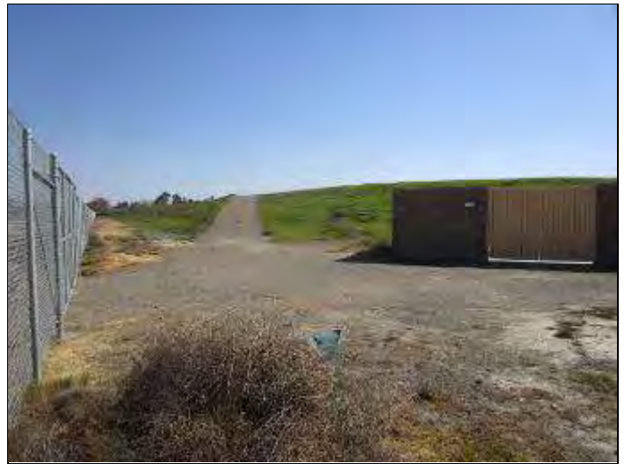
28. Equipment enclosure and driveway to pond south of Parcel 192-020-140
