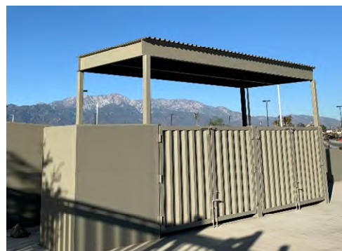
Photo Example 8 Enclosed refuse areas
