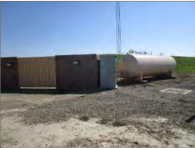
27. Pond, water tank, and pump equipment south of Parcel 192-020-140
