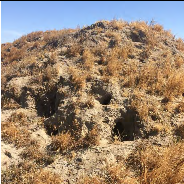
7. Looking east at a large upland berm with a network of ground squirrel burrows. Photo May 7, 2021.
