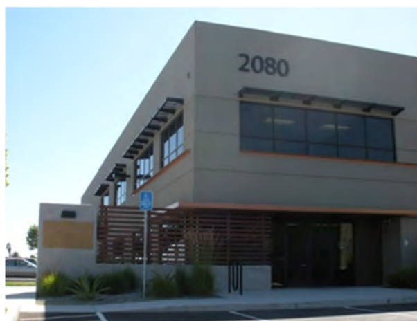
Photo Example 18 Entry protected from the elements.
