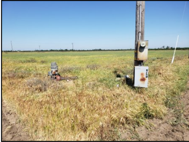
17 : Photograph of abandoned water well and electric service meter located in southeast corner of subject property.
