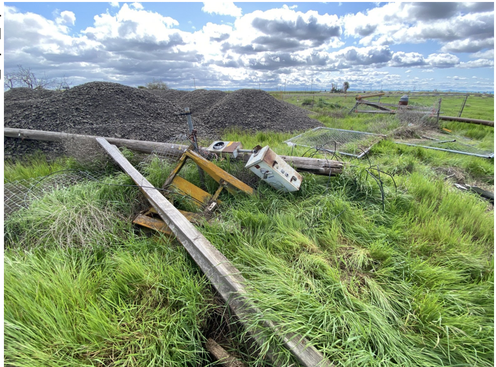
Photo 12: Former electrical equipment located northeast of former residence. View looking south.
