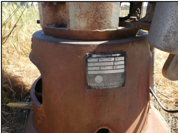
15 : Photograph of abandoned water well located in southeast corner of subject property.
