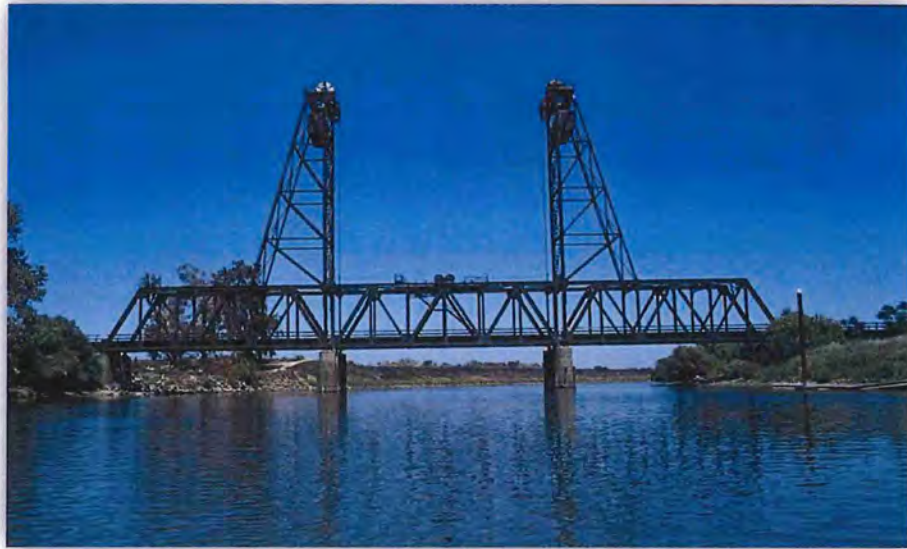
Lathrop – Mossdale Bridge
