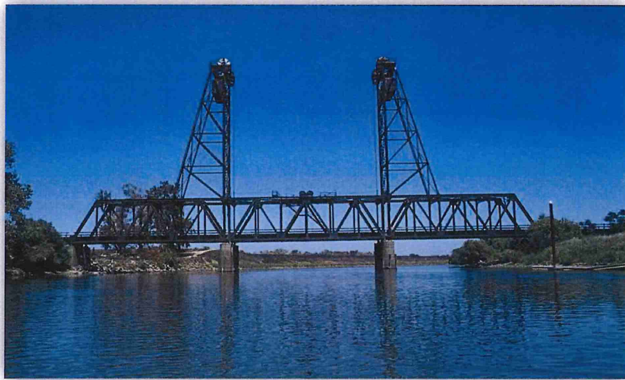
Lathrop – Mossdale Bridge
