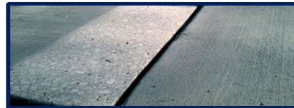
ADA Compliant Trip Hazard Repair
