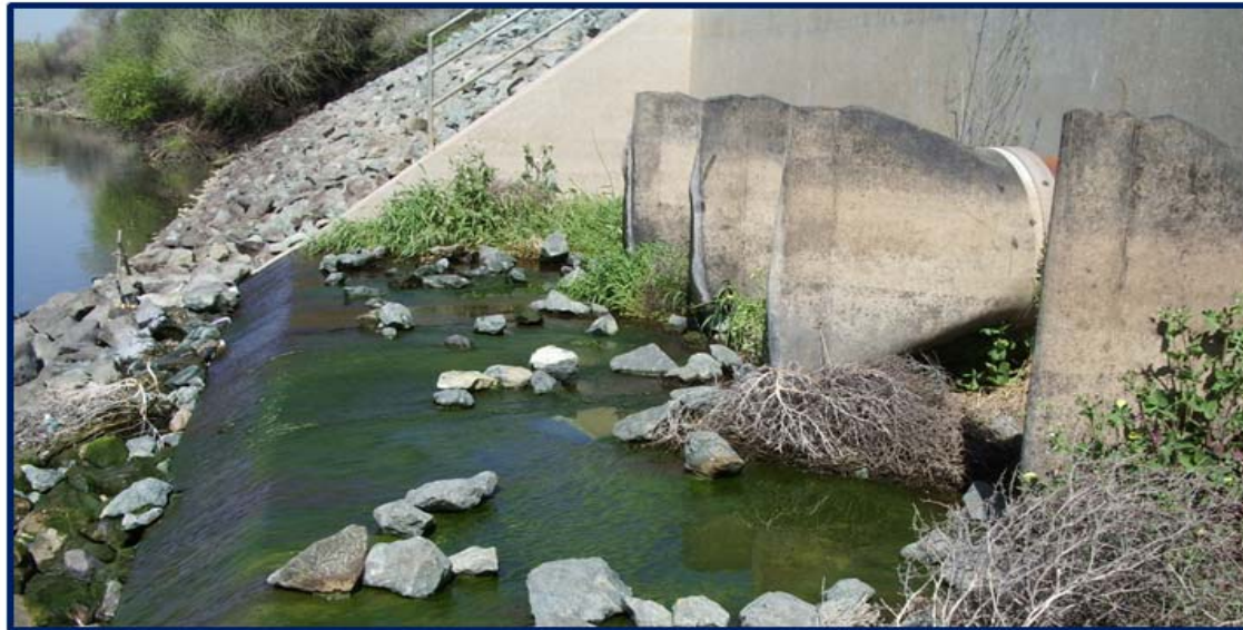
Mossdale Storm Water Outfall to the San Joaquin River
