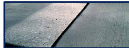
ADA Compliant Trip Hazard Repair
