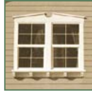
Sill with corbels
