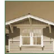
Decorative gable-end detailing
