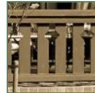
Cut out panels
