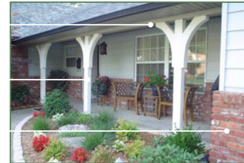
Single hung windows with mullions Wood post with bracket Brick accent material
