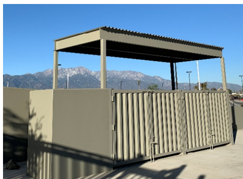
Photo Example 8 Enclosed refuse areas
