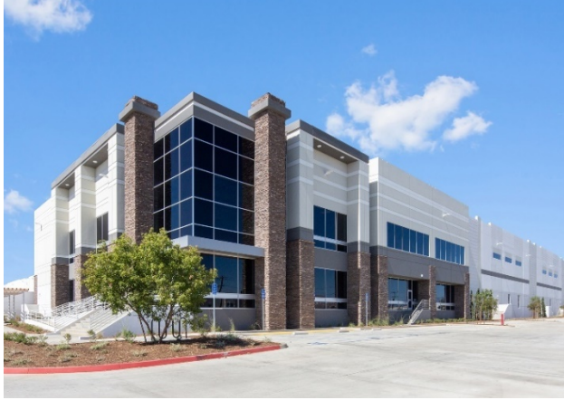
Photo Example 19 Architectural points of interest at entryways
