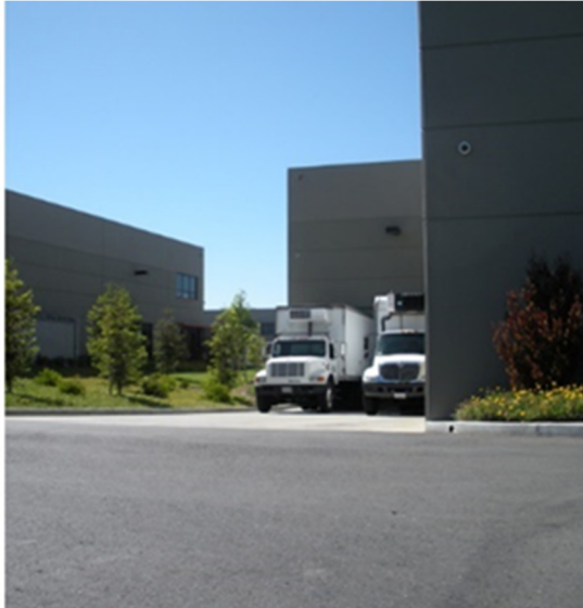
Photo Example 6 Sufficiently sized loading docks
