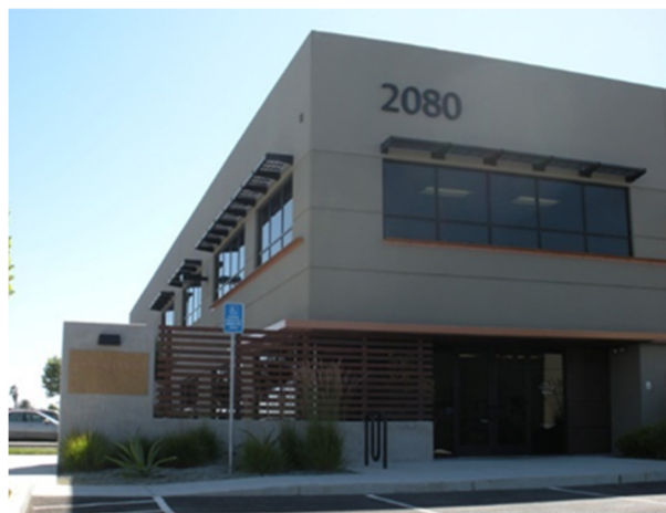
Photo Example 18 Entry protected from the elements.
