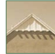
Decorative gable detailing
