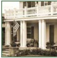
Double wide wood posts
