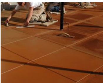
Colored Concrete w/ Pattern
