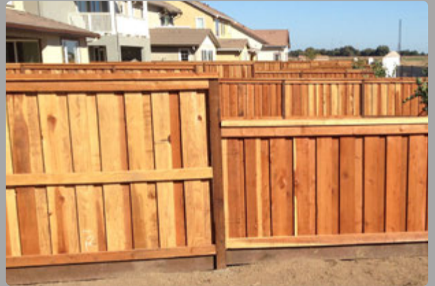
5' to 6' Lake Front Transition Fence
