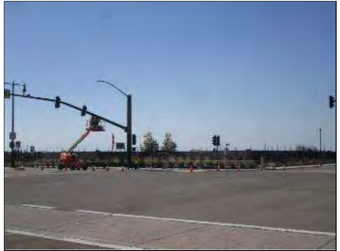
20. Intersection of Spartan Way and Golden Valley Parkway and vacant land south of Spartan Way
