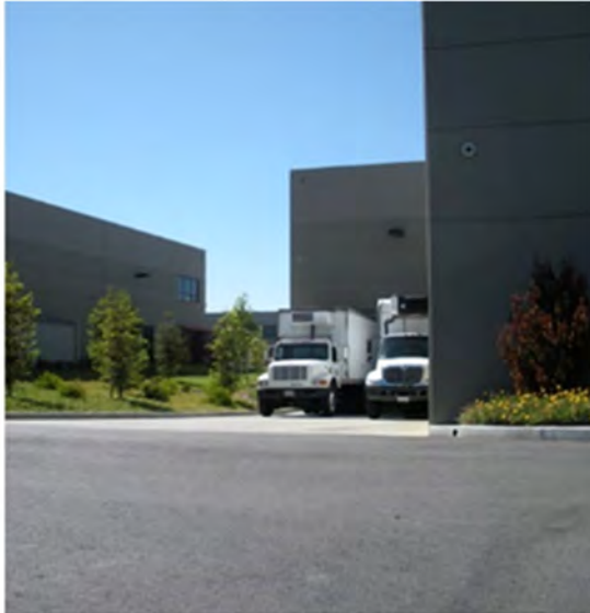
Photo Example 6 Sufficiently sized loading docks
