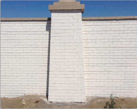
8' Tall Masonry Column with 6' Community Masonry Wall
