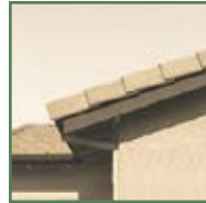
Chamfered rafter tails
