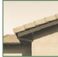
Chamfered rafter tails
