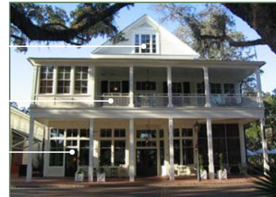
Single hung windows with mullions
