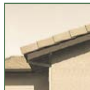
Chamfered rafter tails
