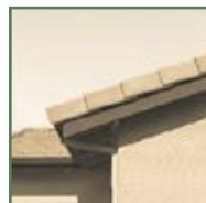
Chamfered rafter tails
