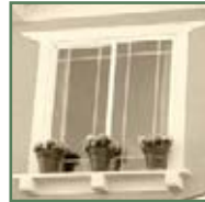
Sill with corbels
