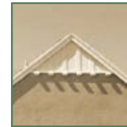
Decorative gable-end detailing
