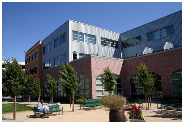
Photo Example 15 Employee well-being area
