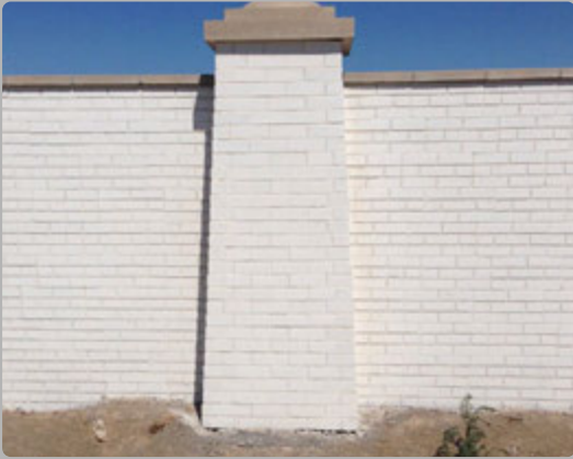
8' Masonry Column with 6' Community Masonry Wall
