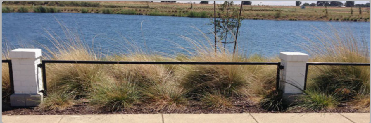
Open Space Rail Fence
