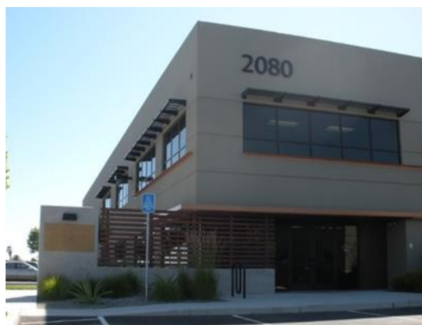
Photo Example 18 Entry protected from the elements.
