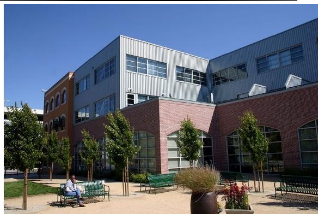
Photo Example 15 Employee well-being area
