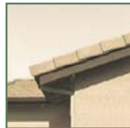
Chamfered rafter tails
