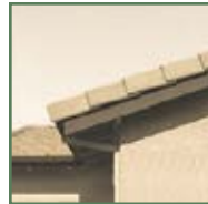
Chamfered rafter tails
