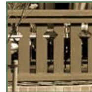
Cut out panels
