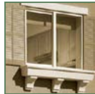
Sill with corbels
