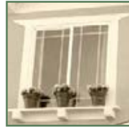
Sill with corbels
