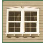
Sill with corbels
