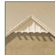
Decorative gable-end detailing
