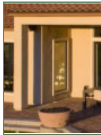
Square stucco columns
