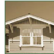
Decorative gable-end detailing
