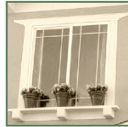
Sill with corbels
