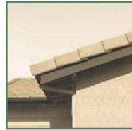
Chamfered rafter tails
