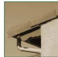
Shaped rafter tails
