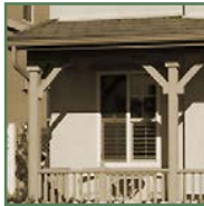
Wood post with bracket 6" min.
