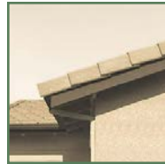
Chamfered rafter tails
