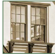
Sill with corbels
