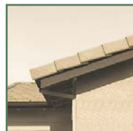
Chamfered rafter tails
