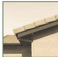
Chamfered rafter tails
