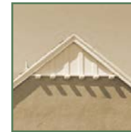
Decorative gable-end detailing
