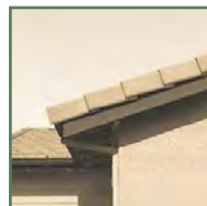
Chamfered rafter tails
