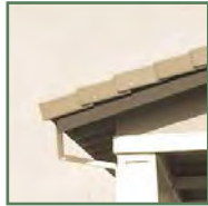
Square rafter tails
