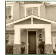
Decorative gable-end portal
