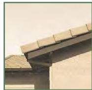
Chamfered rafter tails
