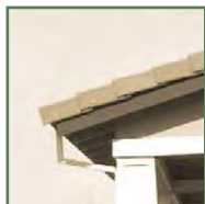
Square rafter tails
