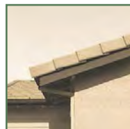
Chamfered rafter tails
