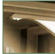
Corbel to fascia
