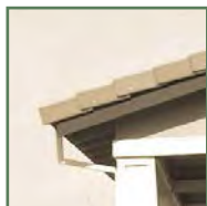
Square rafter tails
