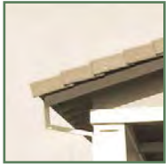
Square rafter tails
