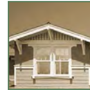
Decorative gable-end detailing
