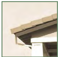
Square rafter tails
