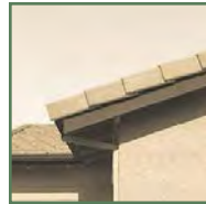
Chamfered rafter tails
