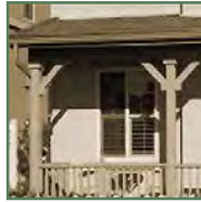
Wood post with bracket 6" min.
