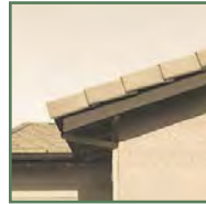
Chamfered rafter tails
