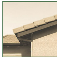
Chamfered rafter tails
