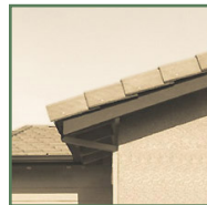
Chamfered rafter tails
