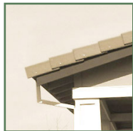
Square rafter tails
