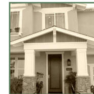
Decorative gable-end portal
