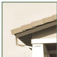
Square rafter tails
