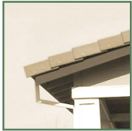
Square rafter tails
