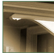
Corbel to fascia
