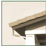
Square rafter tails
