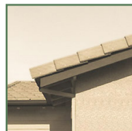
Chamfered rafter tails
