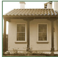
Wood post with corbel 6" min.
