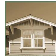
Decorative gable-end detailing
