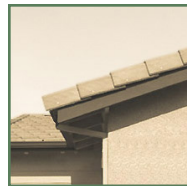
Chamfered rafter tails
