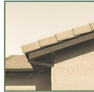
Chamfered rafter tails
