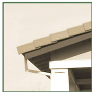
Square rafter tails
