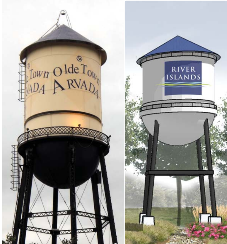
Water Tower Monument with Signage
