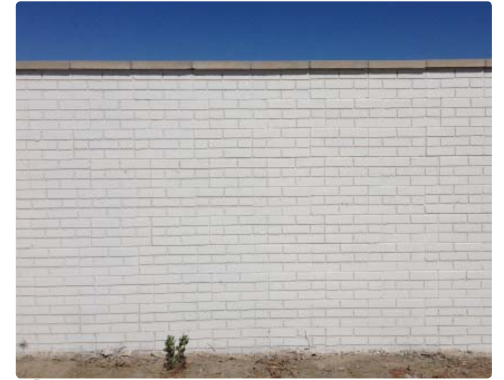
6' Community Masonry Wall
