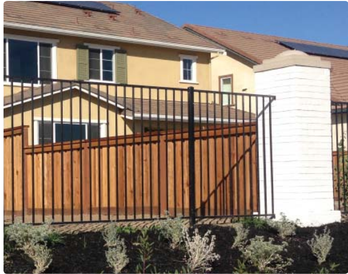
8' Masonry Column with 5' Tubular Steel Fence
