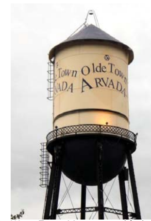
Water Tower Monument with signage
