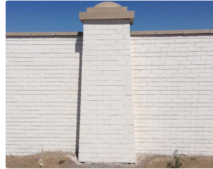
8' Masonry Column with 6' Community Masonry Wall
