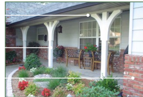
Single hung windows with mullions Wood post with bracket Brick accent material
