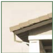
Square rafter tails
