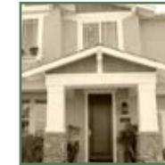
Decorative gable-end portal
