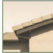
Chamfered rafter tails
