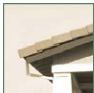
Square rafter tails
