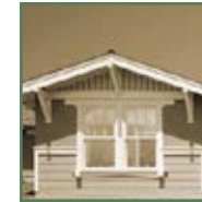
Decorative gable-end detailing
