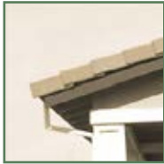
Square rafter tails
