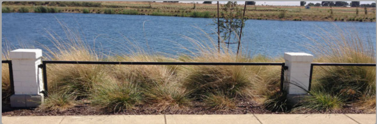
Open Space Rail Fence
