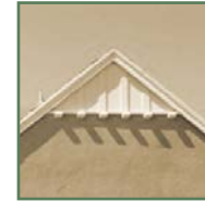
Decorative gable detailing
