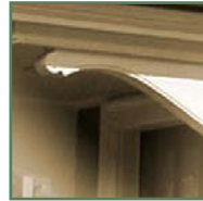
Corbel to fascia
