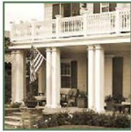
Double wide wood posts
