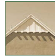
Decorative gable-end detailing
