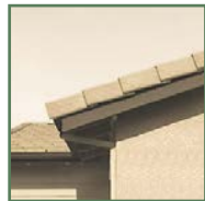
Chamfered rafter tails
