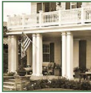
Double wide wood posts
