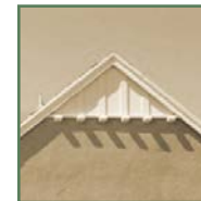
Decorative gable-end detailing
