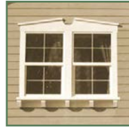
Sill with corbels
