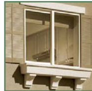
Sill with corbels
