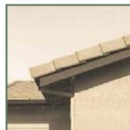
Chamfered rafter tails
