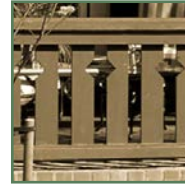
Cut out panels
