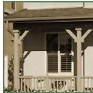
Wood post with bracket 6" min.
