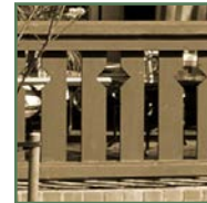
Cut out panels
