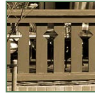
Cut out panels
