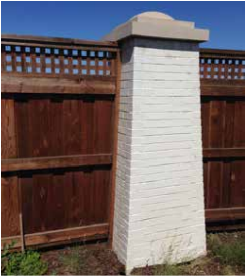
8' Masonry Column with Decorative Wood Community Fence
