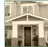
Decorative gable-end portal
