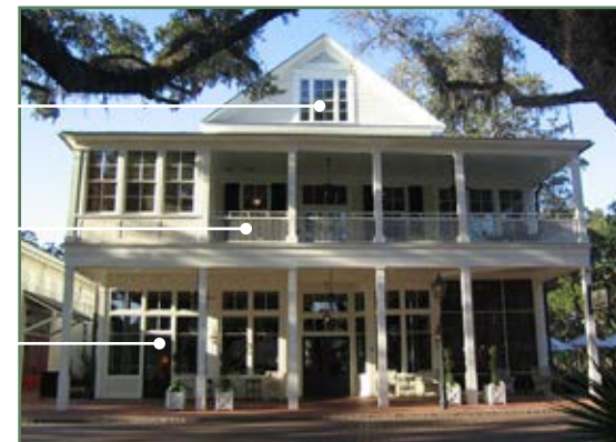
Single hung windows with mullions
