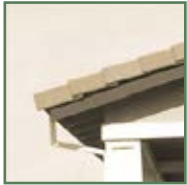
Square rafter tails
