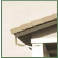
Square rafter tails
