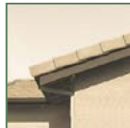
Chamfered rafter tails
