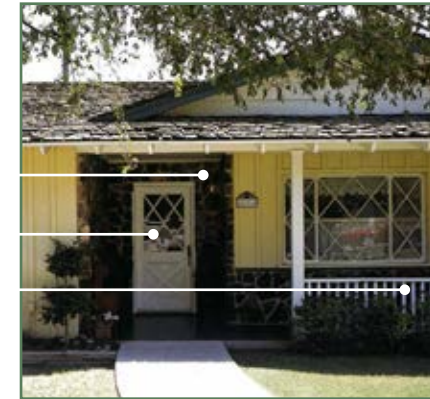
Stone surround Panel door with glass Straight picket railing
