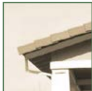
Square rafter tails
