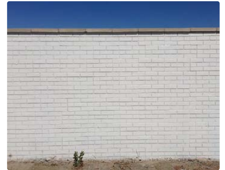
6' Community Masonry Wall
