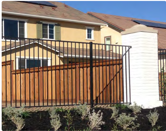
8' Masonry Column with 5' Tubular Steel Fence
