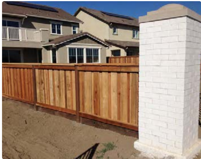
8' Masonry Column with 4' Lake Front Transition Fence
