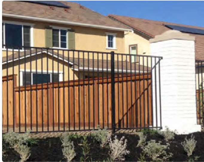
8' Masonry Column with 5' Tubular Steel Fence
