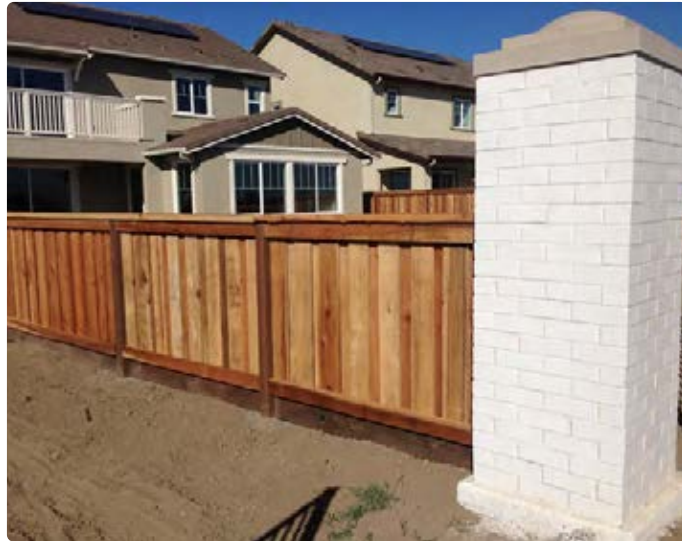
8' Masonry Column with 4' Lake Front Transition Fence
