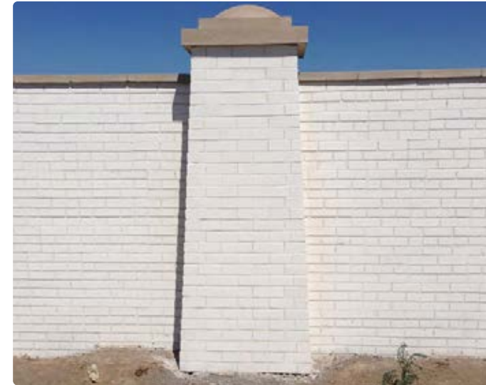
8' Masonry Column with 6' Community Masonry Wall
