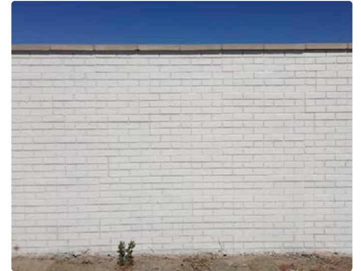
6' Community Masonry Wall
