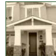
Decorative gable-end portal
