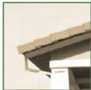
Square rafter tails
