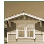
Decorative gable-end detailing
