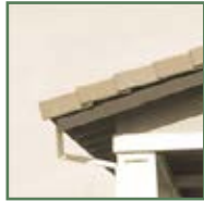
Square rafter tails
