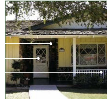
Stone surround Panel door with glass Straight picket railing
