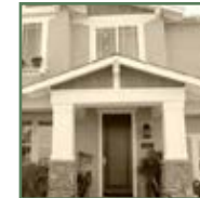
Decorative gable-end portal
