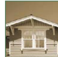
Decorative gable-end detailing
