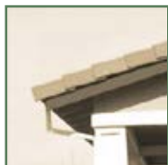
Square rafter tails
