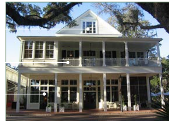
Single hung windows with mullions
