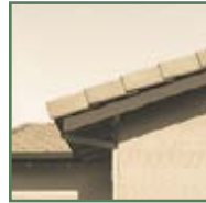
Chamfered rafter tails
