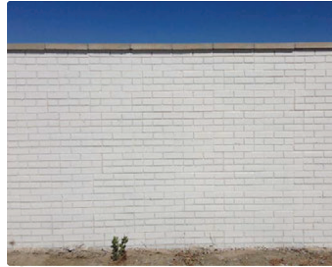
6' Community Masonry Wall
