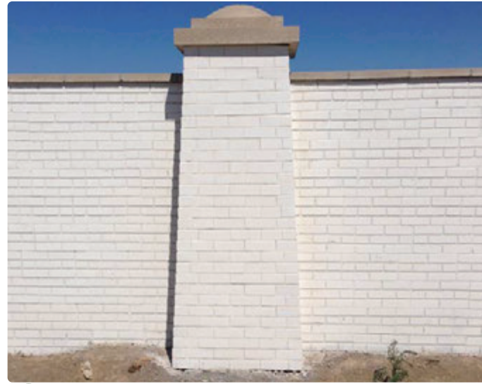
8' Masonry Column with 6' Community Masonry Wall
