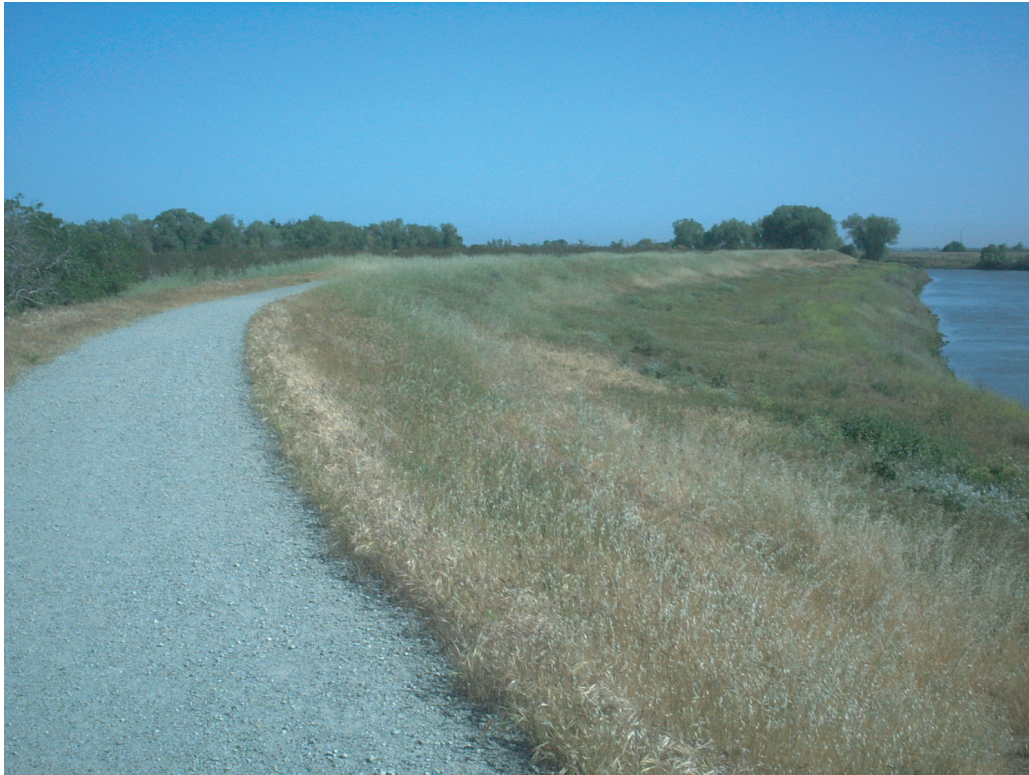
Viewpoint 3: San Joaquin River levee face
