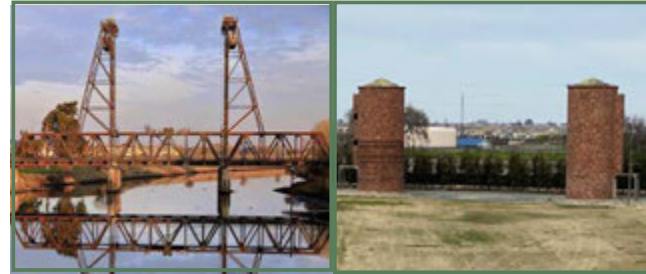
Union Pacific Railroad Bridge
