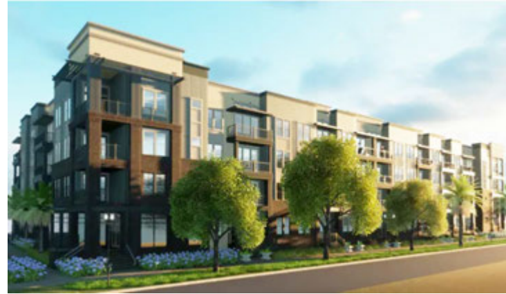
Typical streetscape planting along multi-family buildings
