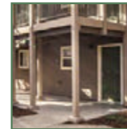
Exposed Wood Column
